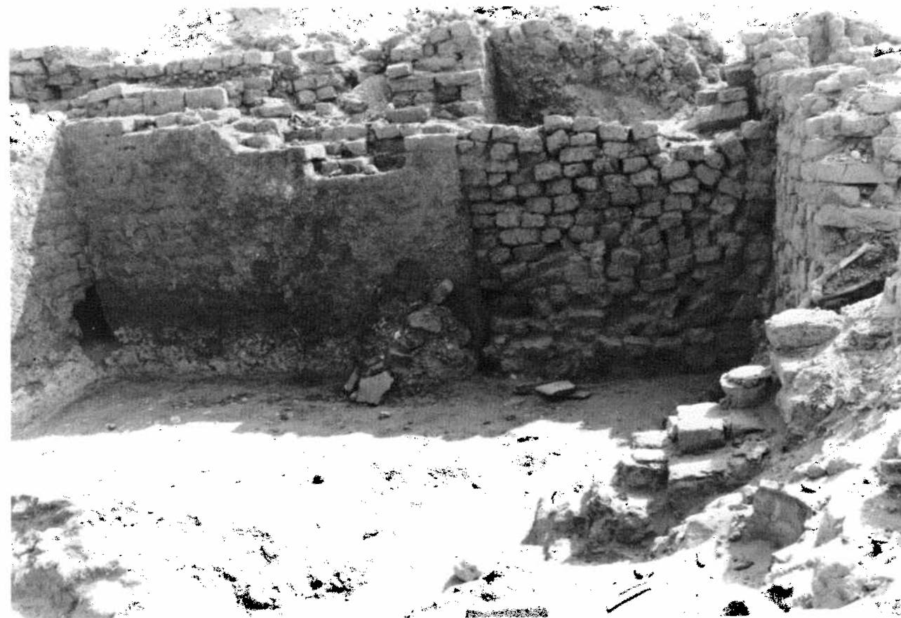
2. Dry masonry brick wall between south balcony (left) and south extension of the platform (right).
