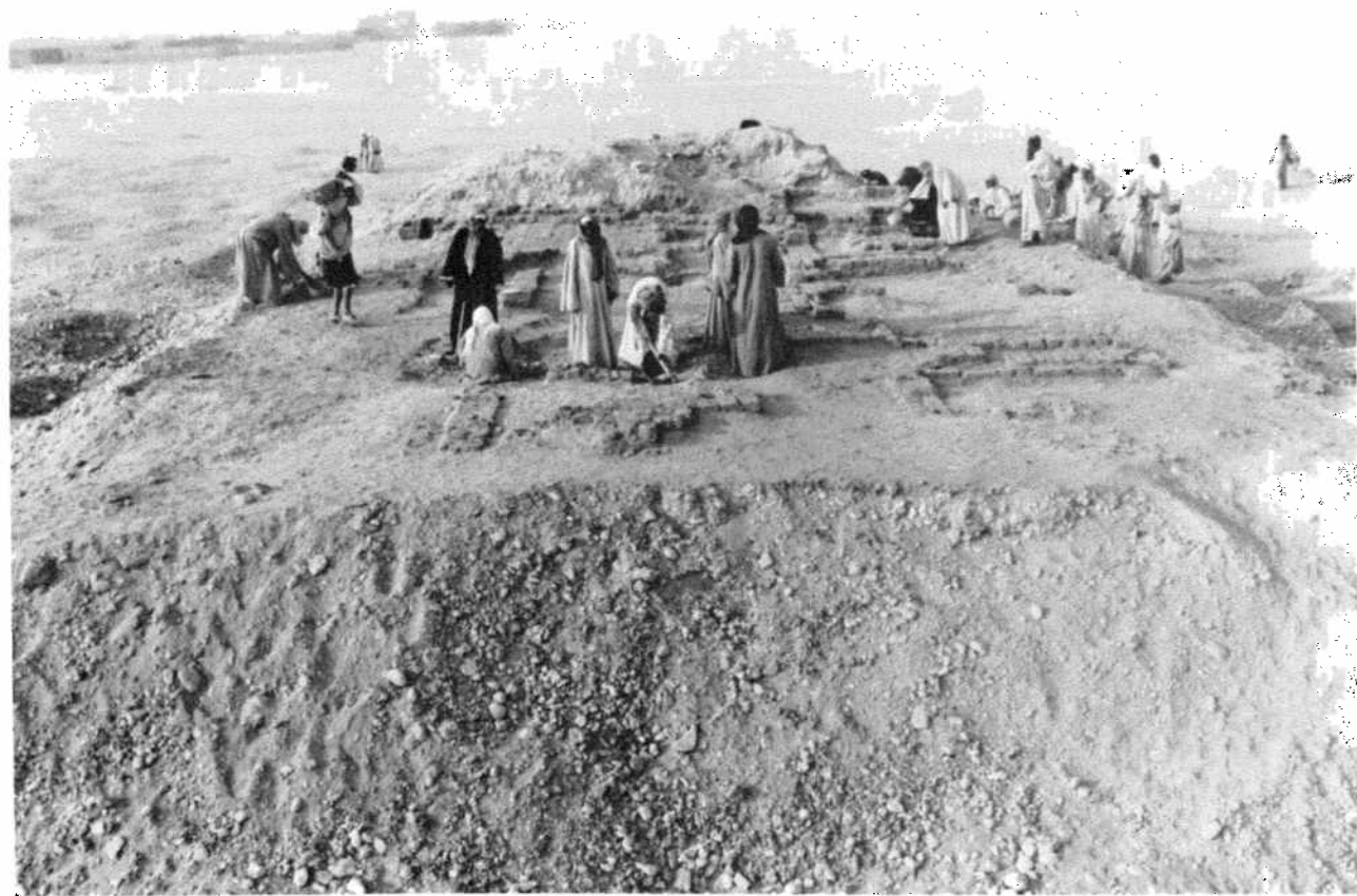
1. Central platform, the work of cleaning.
