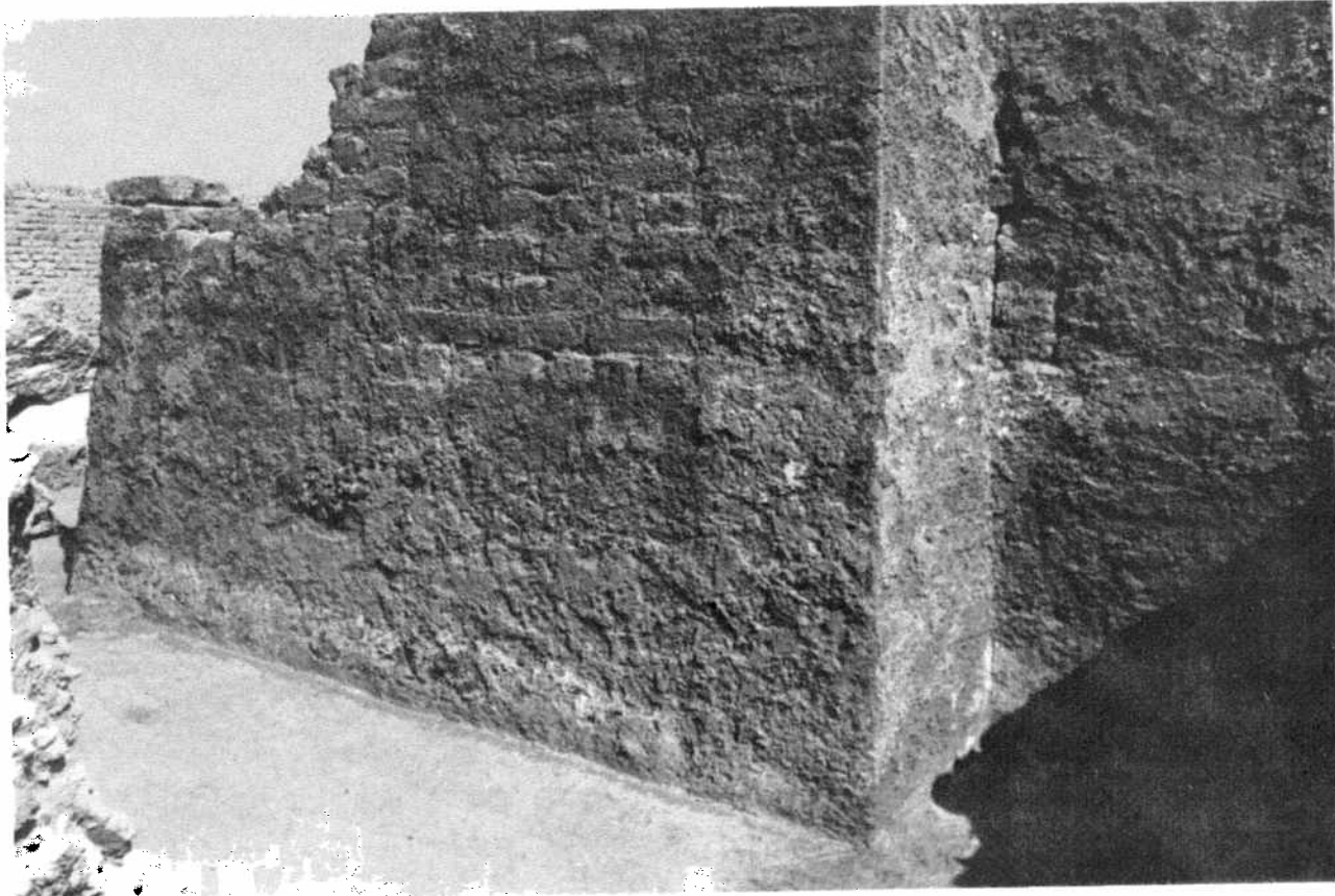
1. Retaining wall of the south balcony.
