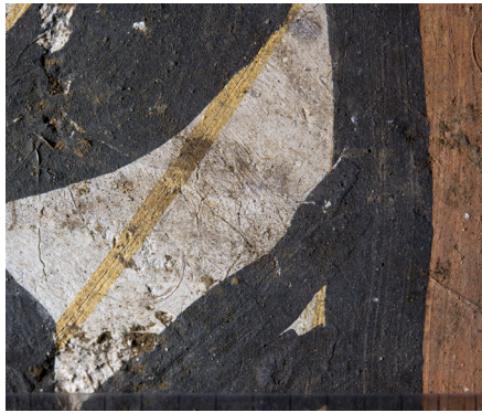
Fig. 17: White lime plaster surface (see Fig. 14) with fine smoothing structures. The yellow paint was applied while the plaster was still slightly damp and plastic leaving brush scratches. Pastose black and red applications apparently followed with an additional organic binder.
